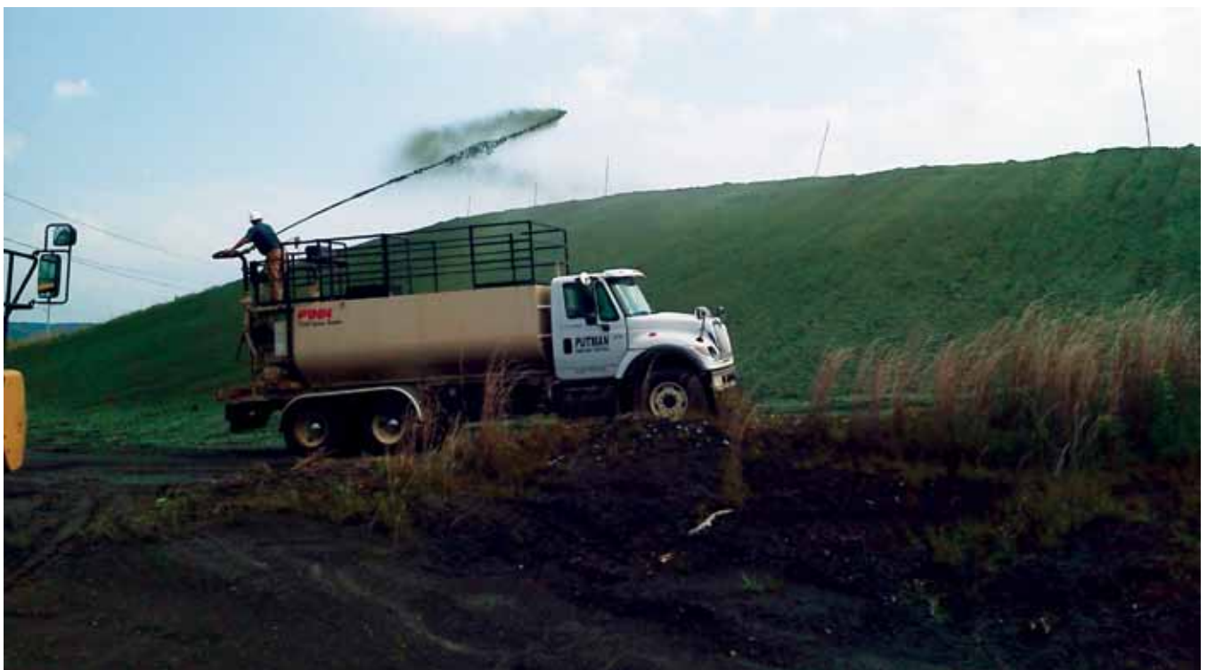
Hydraulic erosion control products are applied as a slurry and engineered to reduce soil erosion while assisting in the establishment and growth of vegetation.
