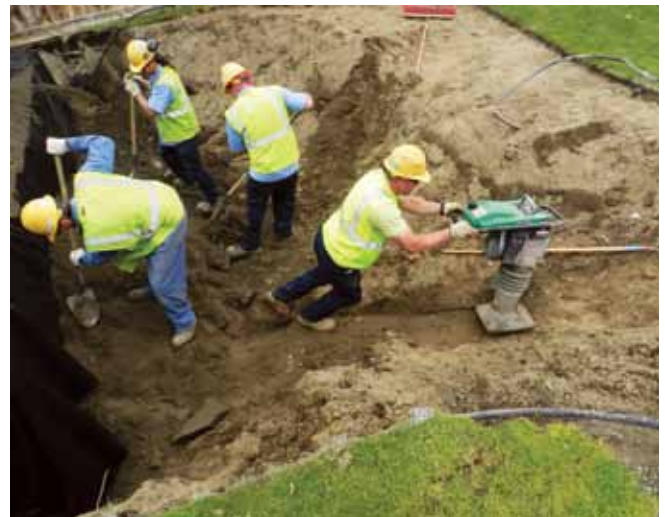
Left: After a flood during an early summer storm in 2011, residents of Spokane incurred damage to their fencing and erosion of their backyards. Right: The construction crew of Spokane's Wastewater Department decided to extend the swale and build cascading steps to control future floods.
