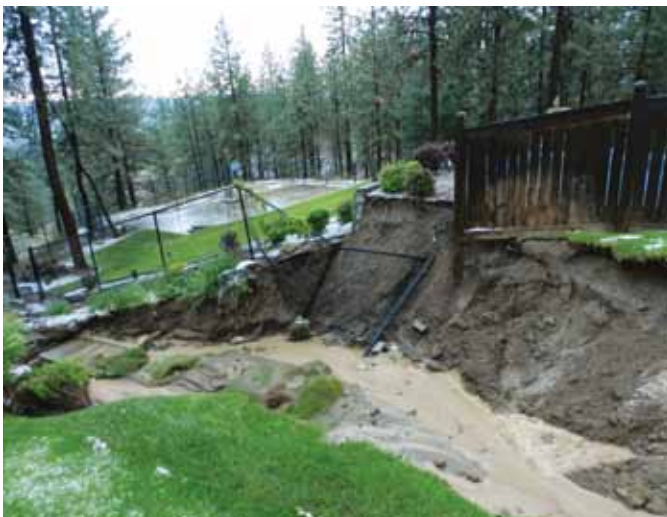
Left: After a flood during an early summer storm in 2011, residents of Spokane incurred damage to their fencing and erosion of their backyards. Right: The construction crew of Spokane's Wastewater Department decided to extend the swale and build cascading steps to control future floods.
