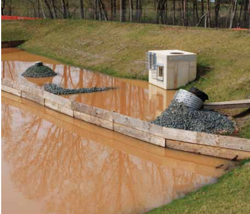
The project basins had various levels of contaminated effluent before Hanes Geo and HaloKlear were called in.
