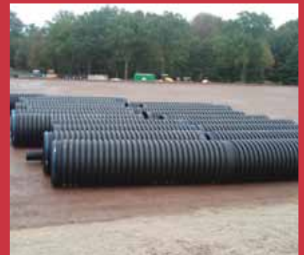
Left: The ground of the athletic field was still damp when work began, meaning no heavy equipment could be used to transport pipe. Right: 60-in. perforated corrugated HDPE and manholes were installed to collect the water and convey it to a detention system.
