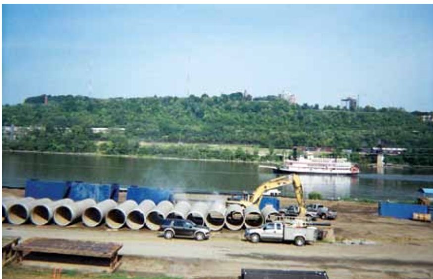
Sections of pipe are lined up awaiting installation.
