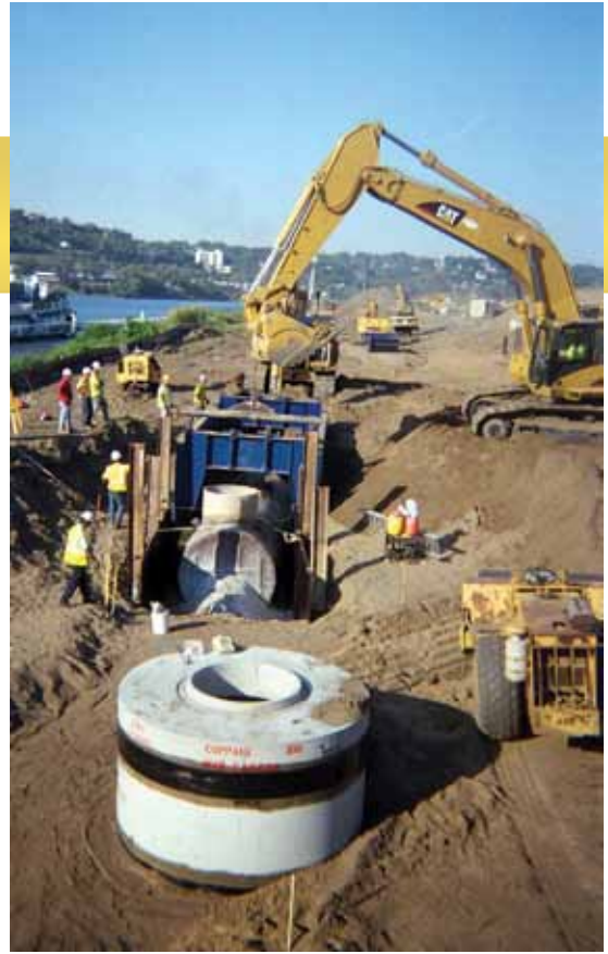
A large-diameter T-base manhole installed near the Ohio River.
