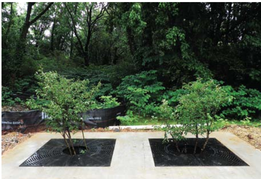
Biofiltration units act as storm drain inlets. They capture suspended solids and pollutants from storm water; the trees, in turn, take in water and nutrients from the runoff.
