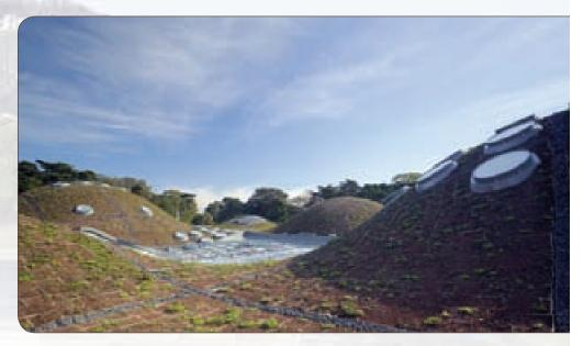
An intricate system of gabion curbs intercepts runoff, preventing erosion.
