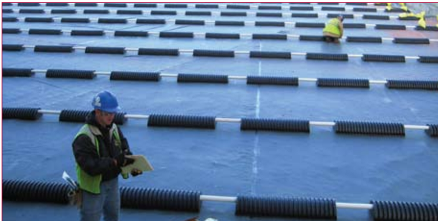
The stadium's storm water system includes a geomembrane liner for erosion control.
