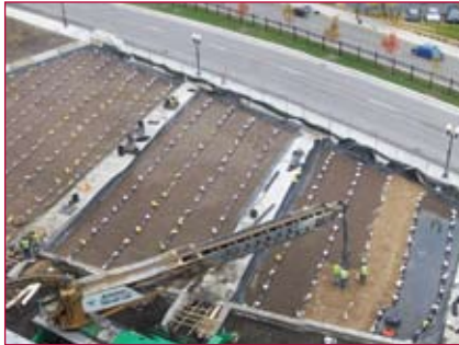
Four workers installed the liner in about five days.
