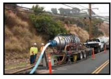
maintain the area's reclaimed water supply during the construction period. Additionally, the work was done within two separate jurisdictions—one that required daytime work and another that required nighttime work. Because Malibu Canyon Road is a two-lane road, often with no shoulder, the work had to be sequenced to minimize traffic impact.
