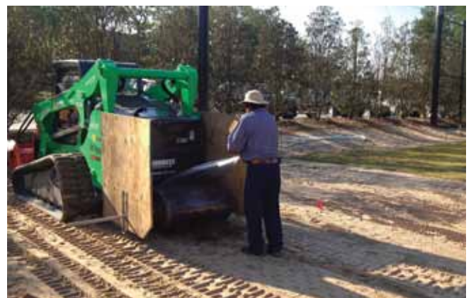
The construction crew used a Blecovator mounted on a skid-steer loader. This machine is a reverse rotating tiller that can break up heavy soils while the leveling bar and roller at the rear of the machine produce a finished grade.
