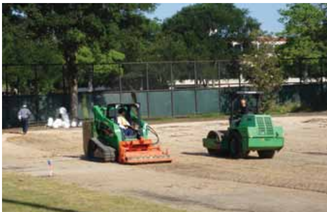
The construction crew used a Blecovator mounted on a skid-steer loader. This machine is a reverse rotating tiller that can break up heavy soils while the leveling bar and roller at the rear of the machine produce a finished grade.
