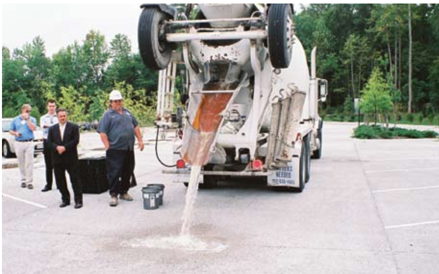
Through pervious concrete infiltration, storm water volume is reduced and pollutants are carried away.
