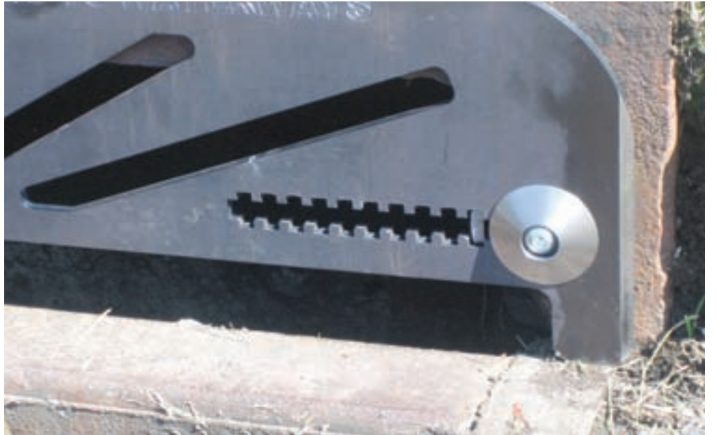
Retrofits are generally mounted to existing catch basin curb heads using a tamper-proof bolt.
