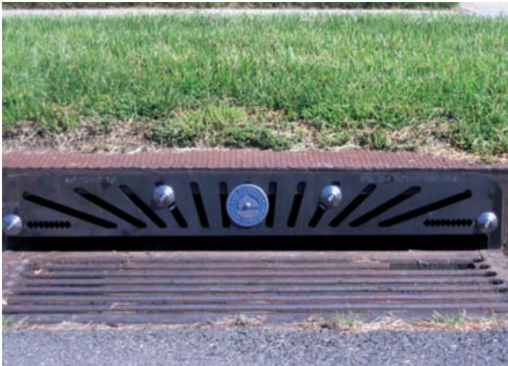
"No Dumping" messages and fish emblems remind residents that what goes down a sewer finds its way to local waterways.
