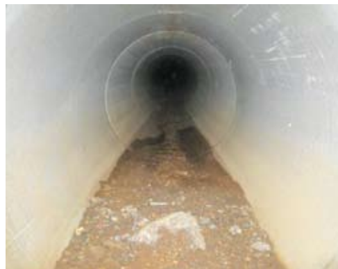
Left: Damage to this water quality device could have been prevented if the catch basins and inlets were protected with hay bales, silt fencing, etc. Right: Storm drain pipe leading to an underground BMP; it is full of debris and should have been jetted out after construction was complete.
