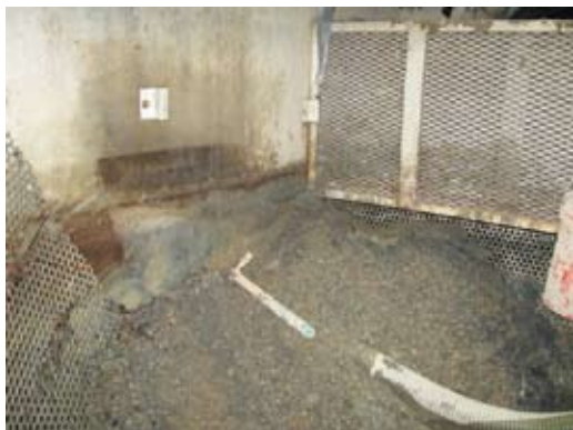
Left: Damage to this water quality device could have been prevented if the catch basins and inlets were protected with hay bales, silt fencing, etc. Right: Storm drain pipe leading to an underground BMP; it is full of debris and should have been jetted out after construction was complete.
