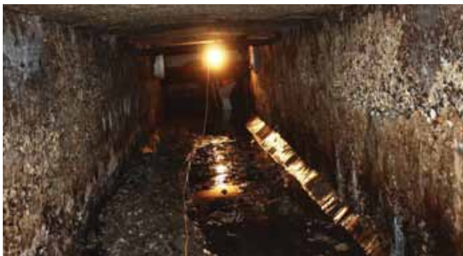
Left: The box culvert under State Road 64 before rehabilitation was believed to be almost a century old and was structurally unsound. Right: After rehabilitation, there are no signs of shrinkage, and the culvert appears watertight.
