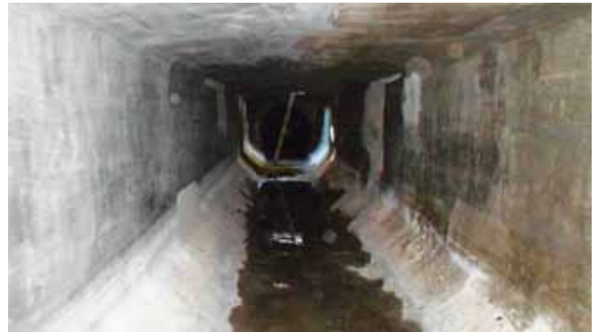
Left: The box culvert under State Road 64 before rehabilitation was believed to be almost a century old and was structurally unsound. Right: After rehabilitation, there are no signs of shrinkage, and the culvert appears watertight.
