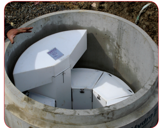
Upflow technologies provide room for filter media to swell and circulate.
