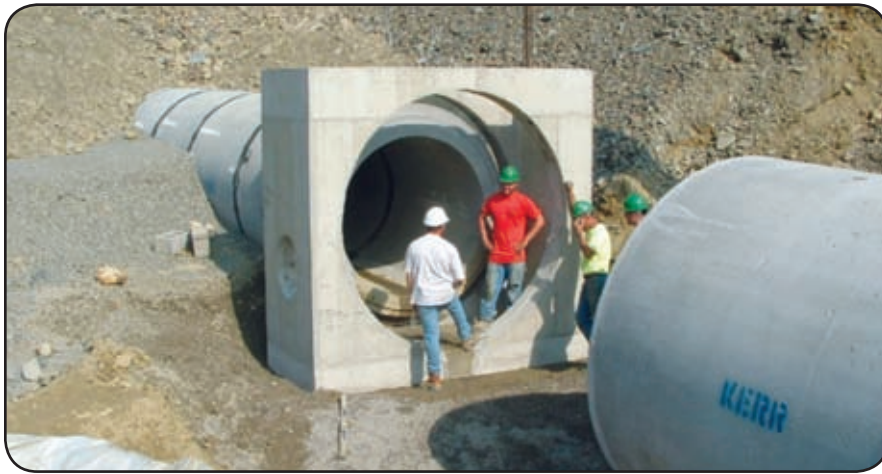
PennDOT has used special design-heavy, wall-reinforced concrete pipe in 10 PAIDD projects.
