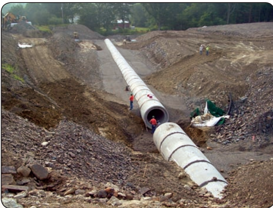
Road improvements aim to alleviate Tioga County’s travel problems.
