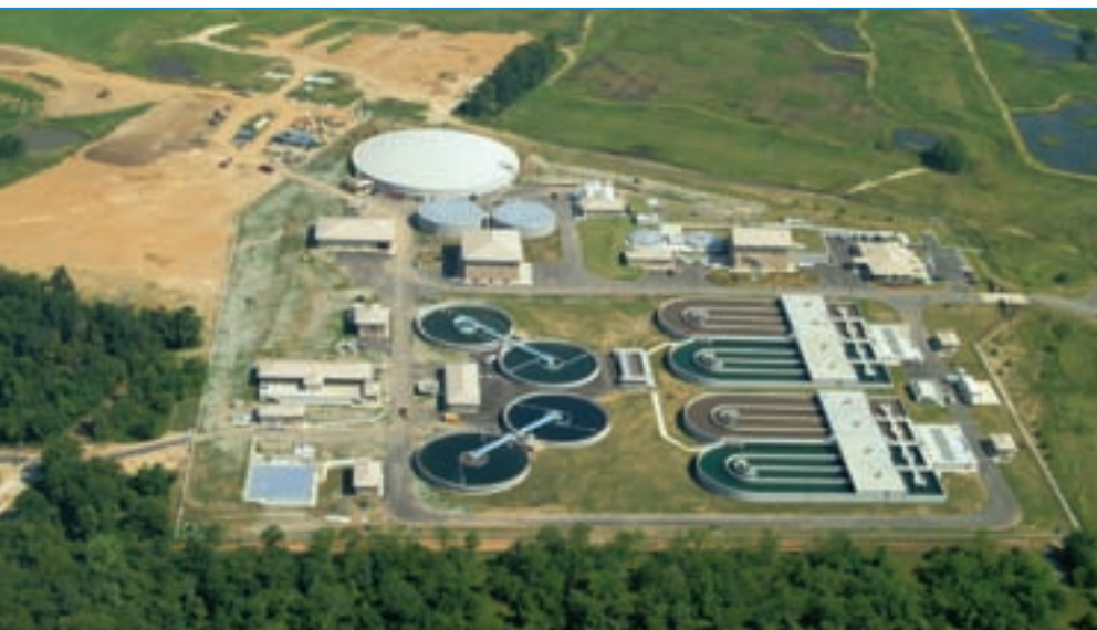
The new Westside WWTP features 46 acres of constructed wetlands.
