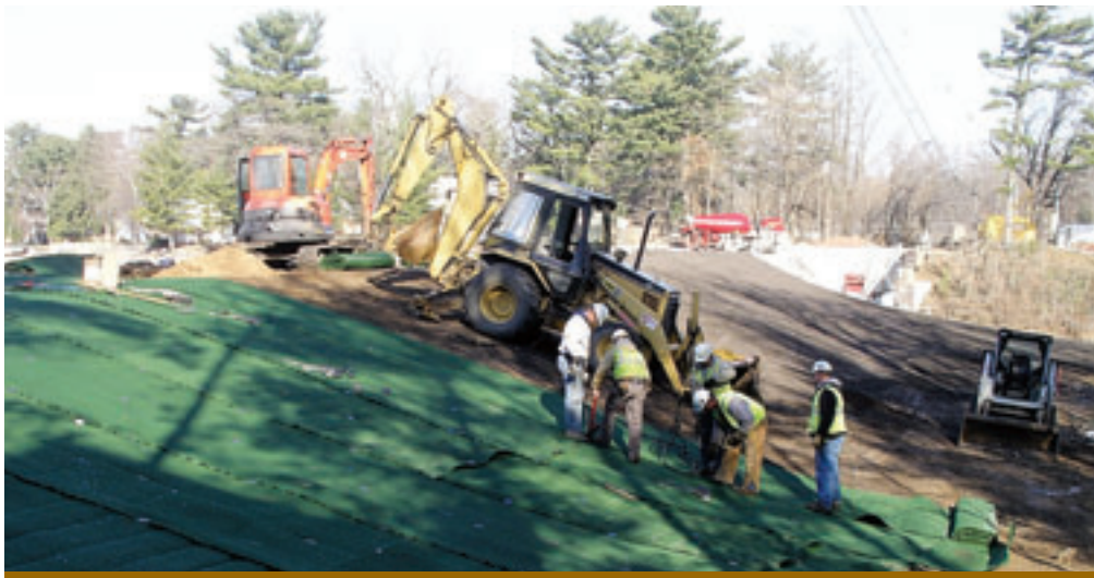
Installation crew members anchored the HPTRM one section at a time.
