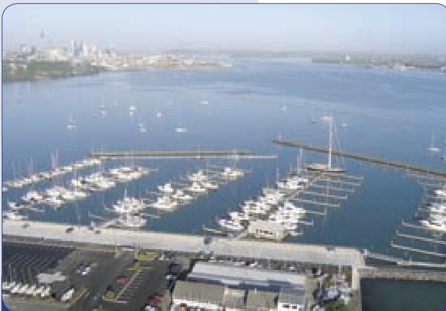
Using upflow technology, New Zealand's Hauraki Gulf surpassed local storm water treatment requirements.
