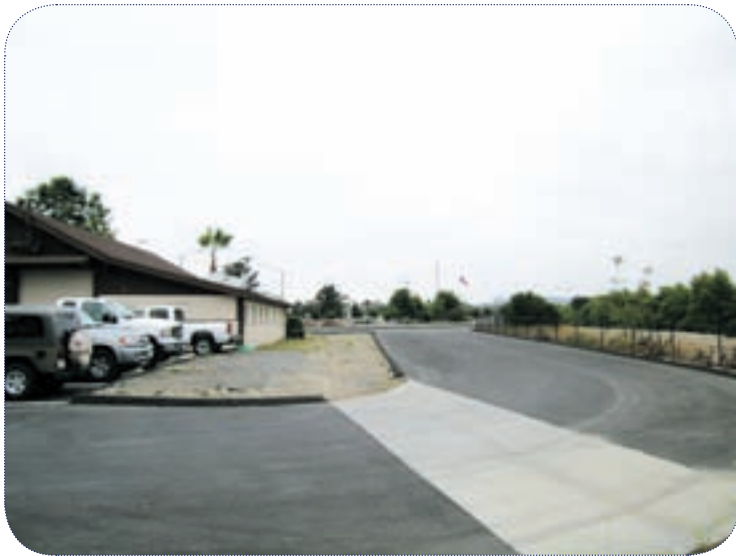
The station's original truck wash area.
