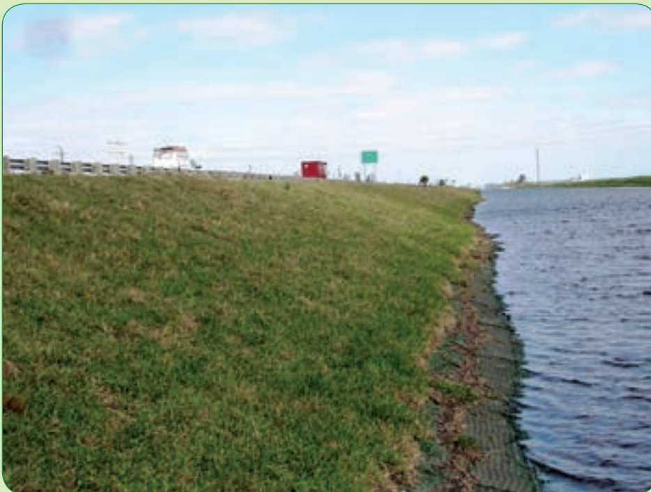
The SFWMD achieved a natural post-construction look on canal C-51.
