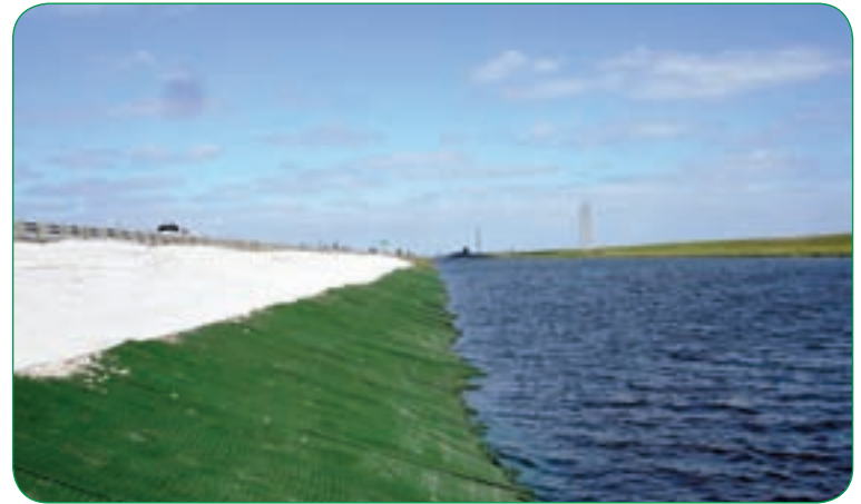
Workers installed approximately 55,000 sq yd of TRMs in about 60 days.
