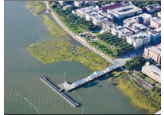
Low-impact design and working landscapes can help restore a site's water balance.
