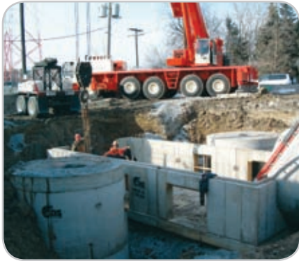
IDOT replaced pumping stations and an automated trash rack with a pair of CDS systems.
