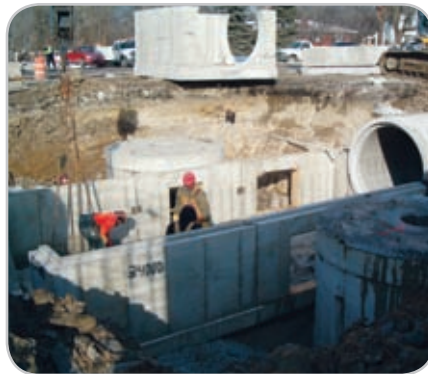
IDOT replaced pumping stations and an automated trash rack with a pair of CDS systems.
