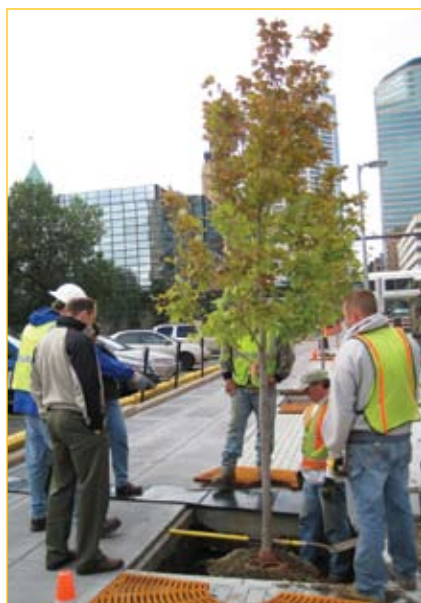
Each of the 179 tree cells installed in downtown Minneapolis can store 134 cu ft of storm water.
