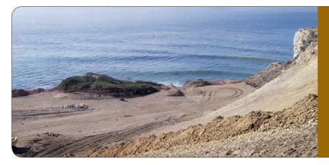
Of three possible repair approaches, project leaders opted to partially remove and rebuild the landward portion of the landslide.
