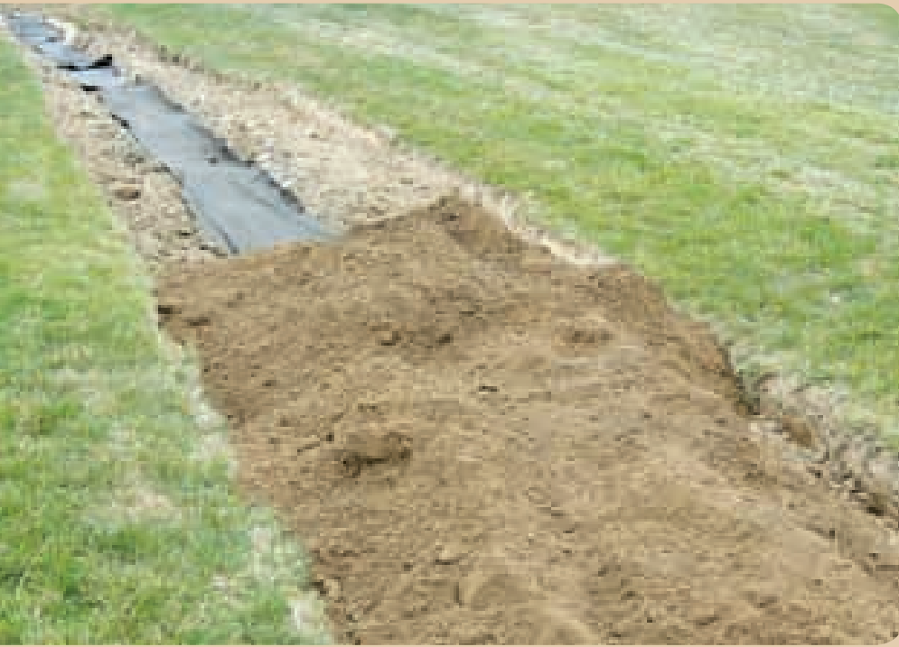
Soil and geotextile cloth topped the drain to complete the upgrade.
