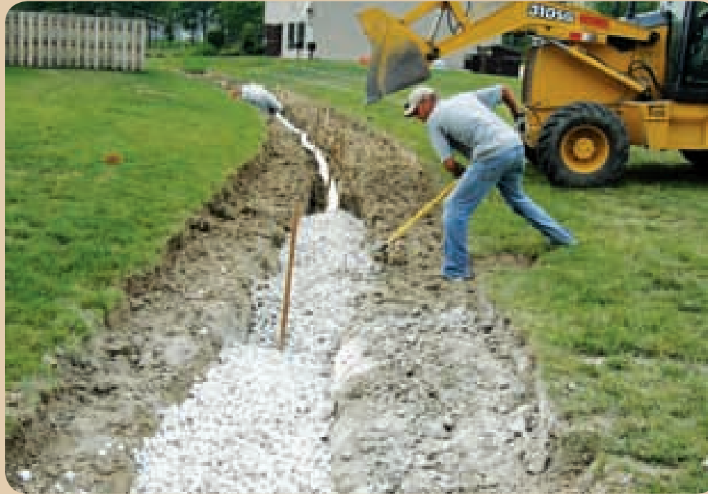
Workers installed stone around the Trailer Transit site's underdrain.
