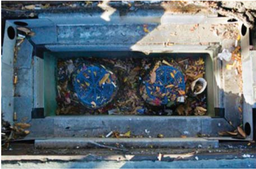
The inserts remove heavy metals, sediment, bacteria, organics, nitrates and litter from storm runoff.
