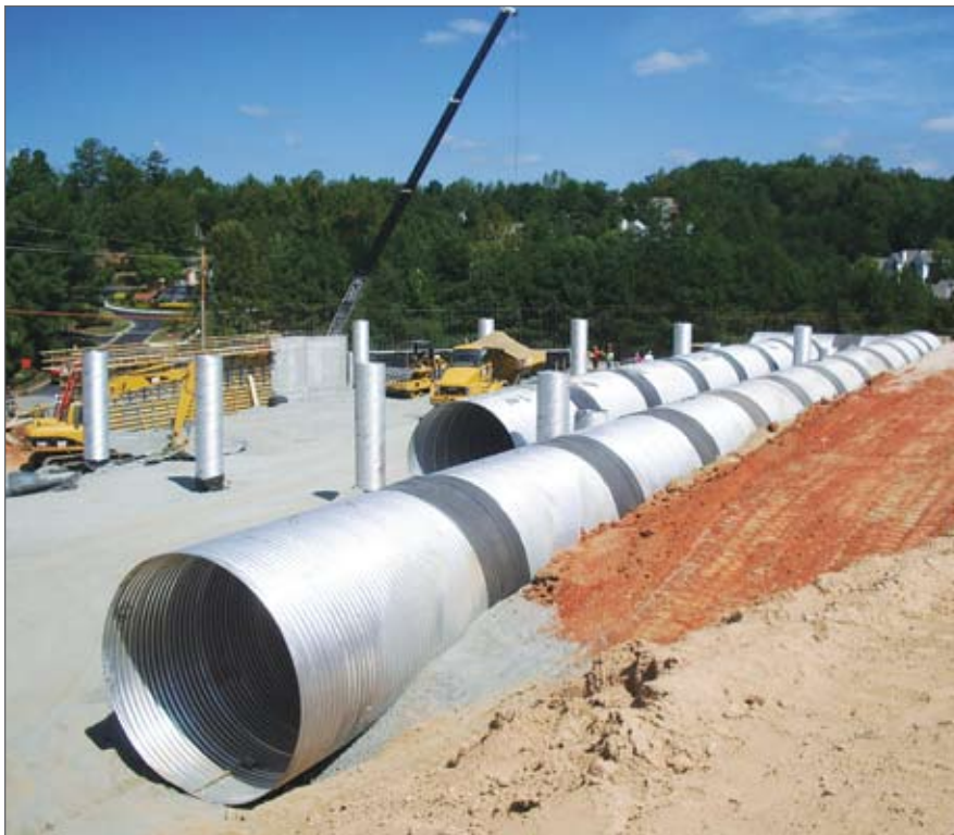
The East Village site required 3,500 ft of 144-in. pipe.
