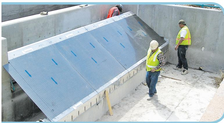
AMAFCA modified a structure on the North Pino Channel using a wedge-wire screen sized to remove all debris and sediment larger than 500 microns. The screen is made up of many triangle-shaped wires that are tilted and welded onto support bars, forming a surface similar to a file, where each wire shears a layer of water.
