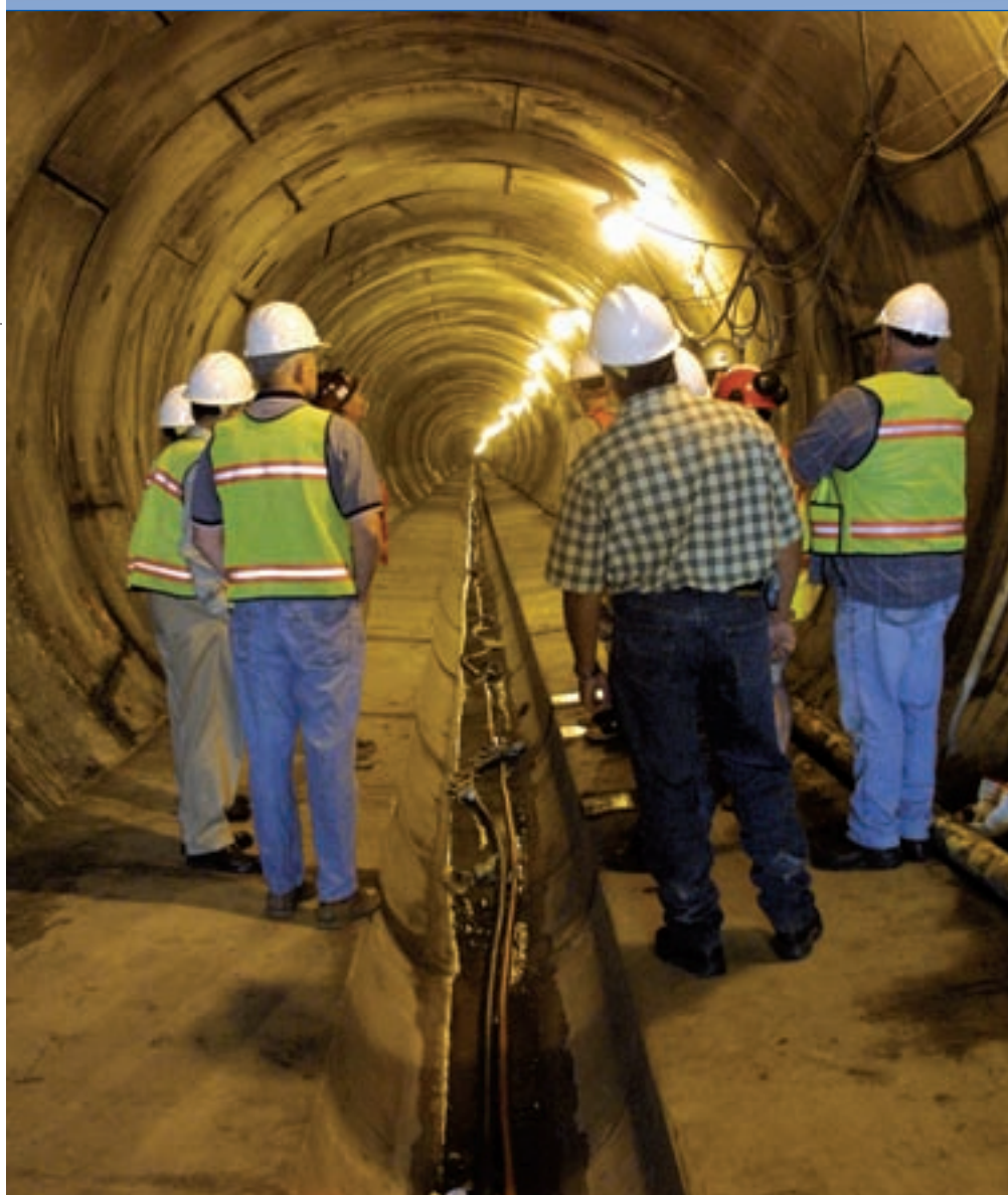
Workers inspect King County's mile-long storage tunnel, completed in 2006.
