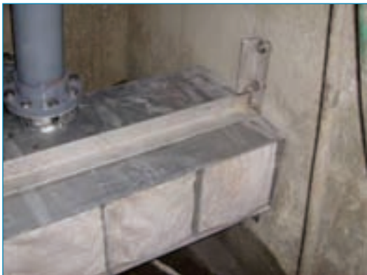
Absorption filter media will treat airport runoff before it is discharged into local waterways.
