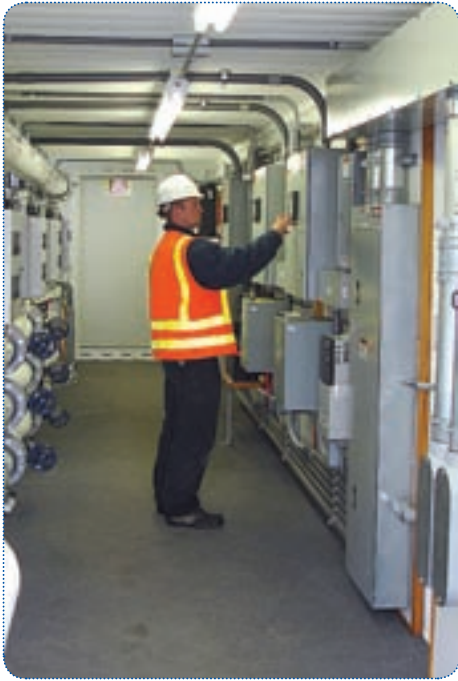
Storm water turbidity, pH and flow are monitored before and after treatment.
