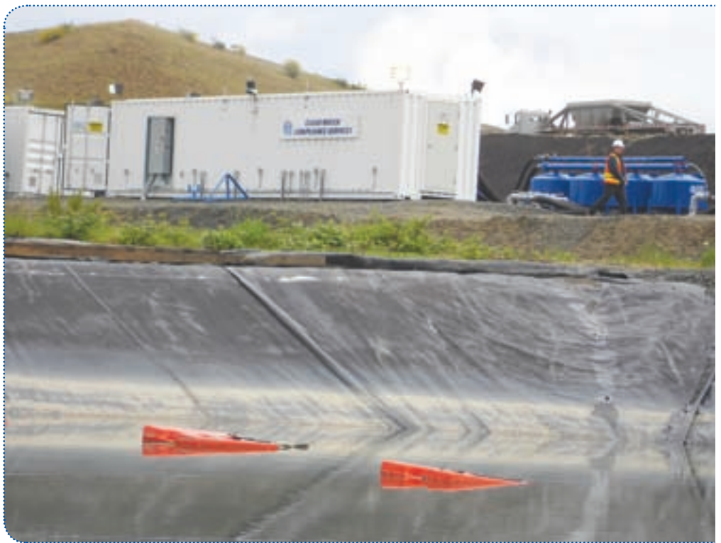
Runoff is collected and stored in four ponds featuring CESF equipment.
