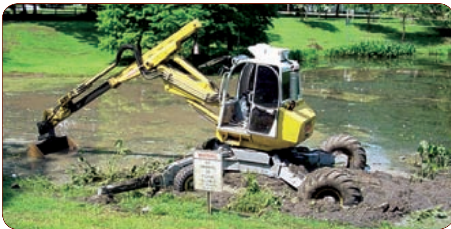
A spreadsheet based on three strategies was used to identify possible BMPs for target watersheds.
