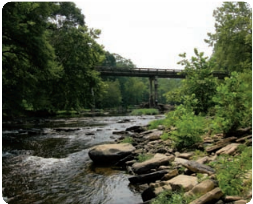
Alabama Bridge Builders constructed this new Blount County bridge over waters containing threatened and endangered species.
