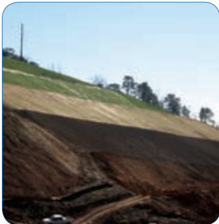
Staged vegetation establishment and benching are used by Wright Brothers in a Talladega County project.
