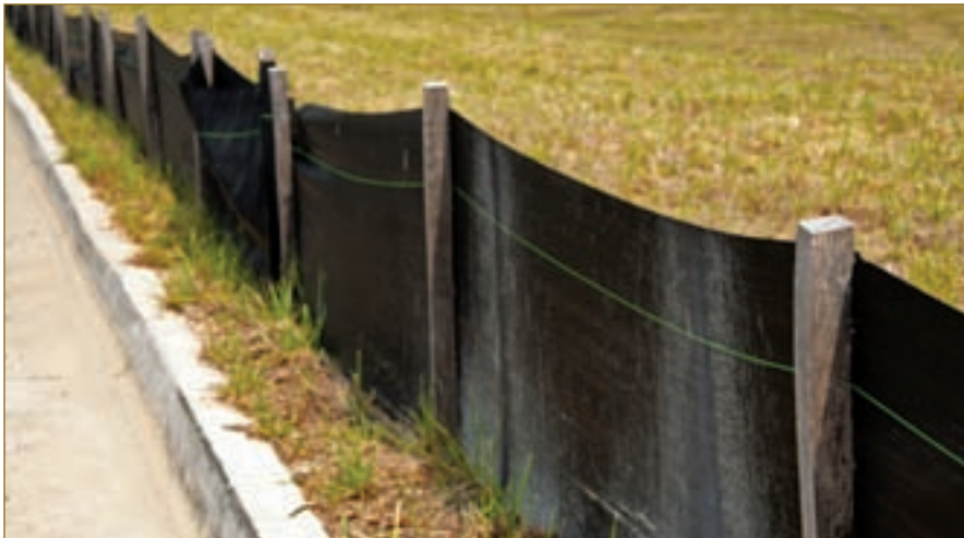
A silt fence is typically 40 to 50 percent effective as a site perimeter sediment control.
