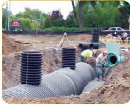
Contractors install water quality units to pretreat retention beds.
